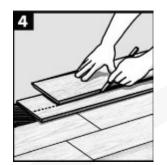
9. Fitting around irregular objects is no problem. Simply make a pattern out of heavy paper to fit around pipes or irregular objects. Place the pattern upon the plank and trace. Cut along trace lines using a utility knife or heavy duty scissors and lay the plank. Be sure to leave a minimum of 1/8" expansion space around all fixed objects, floor vents and door frames.
